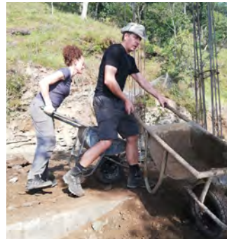
November 2019: Am Fundament
