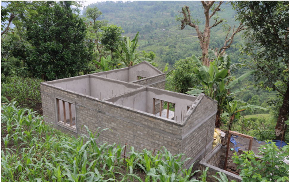
One of the 74 houses. We are getting closer to 108 houses.
