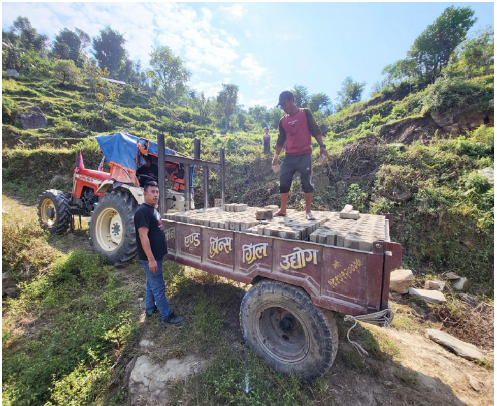
Transport from production to the construction site.
